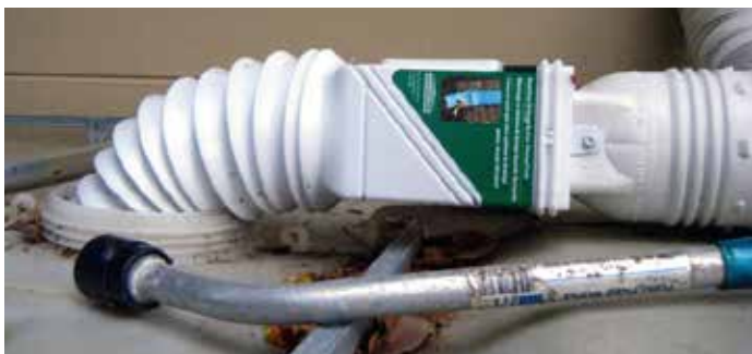
Flexible downspout tubing with debris catcher from gutter to tank
