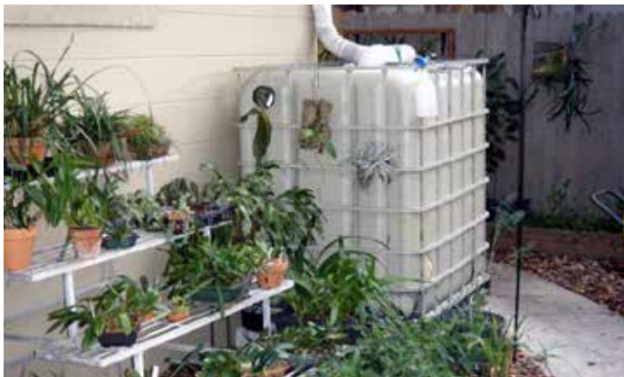
Rainwater collection tank ties into roof downspout
