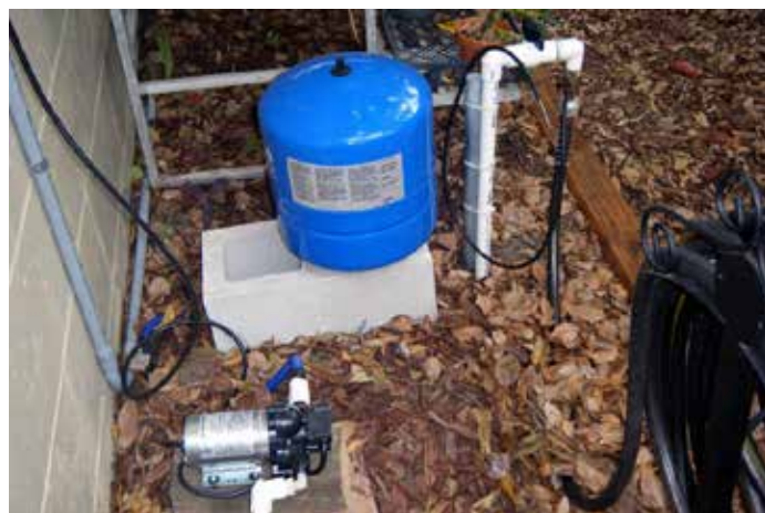
Pump to move water from storage with a bladder tank to help prevent pump from cycling.
